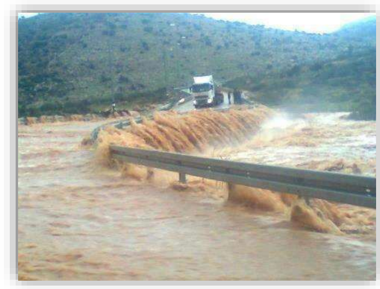
West Bank, 2013 floods
