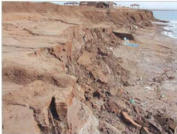
Collapse of sea cliff, 2004 earthquake
