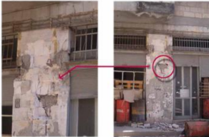
Expulsion of blocks in poor mortar stone
