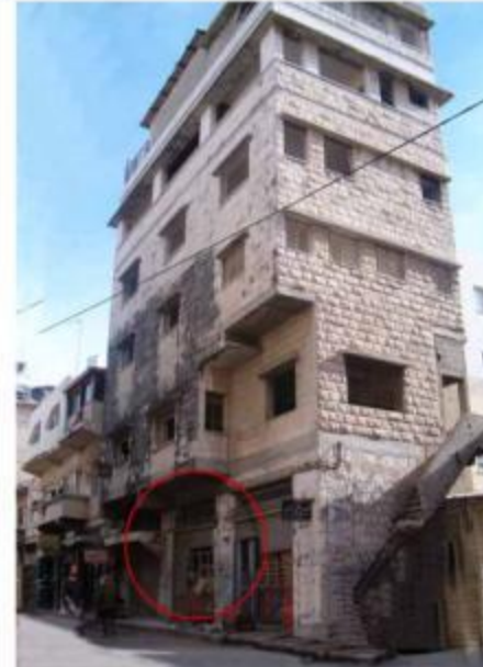
fig.1 Crack Patterns, Crushing and Large permanent deformation in the Masonry Pillars. see more details page no. ( 4/8 )
